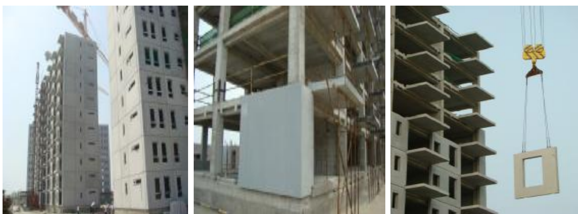
Fig.1 the concrete curtain wall project of Tianjin Vanke Donglihu
