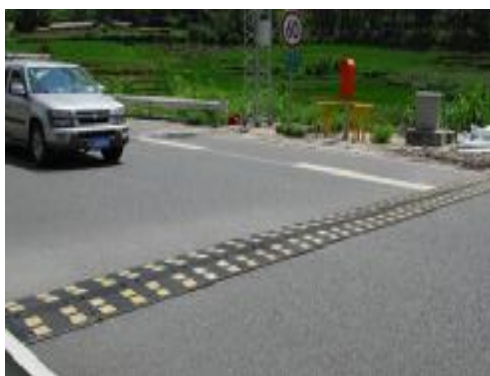
Fig3 vibration acceleration detection on the deceleration zone
