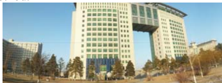
Figure7. After fusion splicing images
