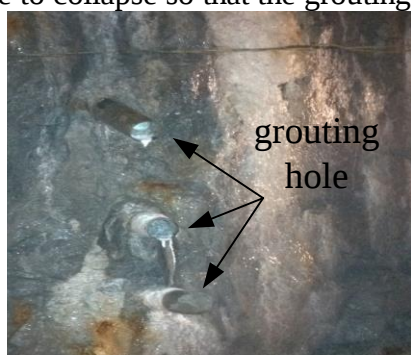
(a) Hole grouting reinforcement
