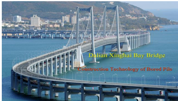
Figure 3. Dalian Xinghai Bay Bridge
