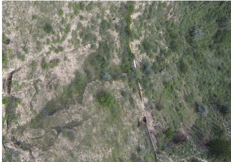
Figure 3. Finite Pipeline image along the mountain
