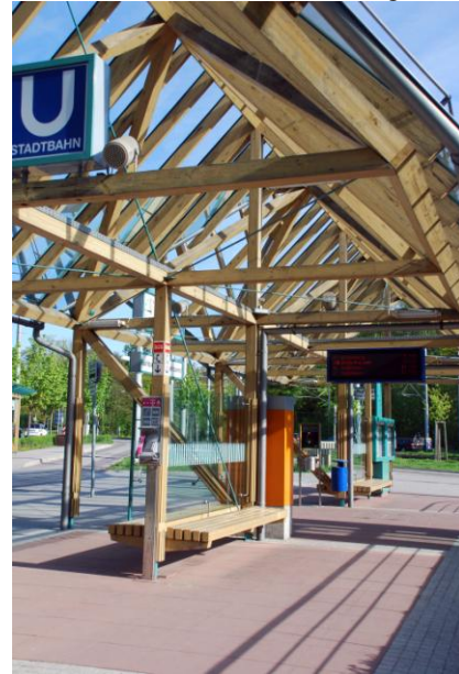
Figure 3. Standardized wood and steel frameworks
