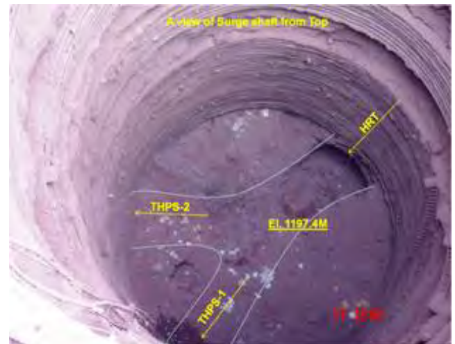
Fig.5 Sinking of Surge Shaft
