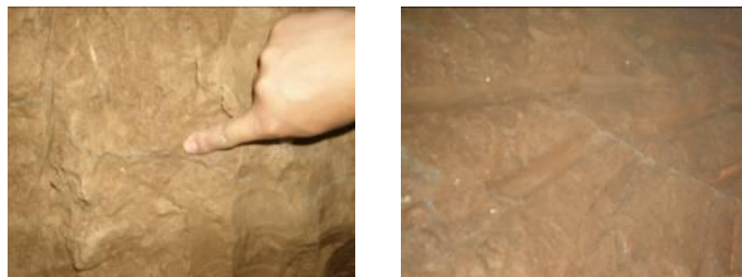
Fig.6 Spot observation of horizontal grouting
