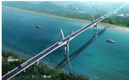
Fig. 2. Extradosed Cable-Stayed Bridge
