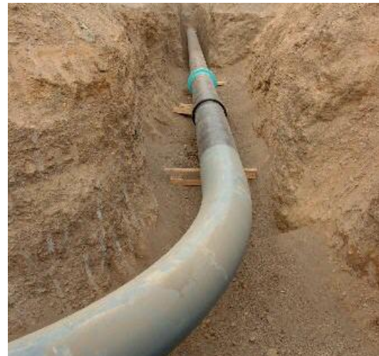
Fig. 1 Buried hot oil pipeline
