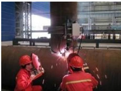
Fig.9 Welding process test
